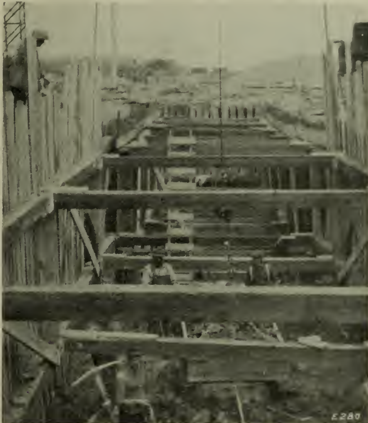
FIG. 2. HAND LABOUR AND WOODEN SKIP.
